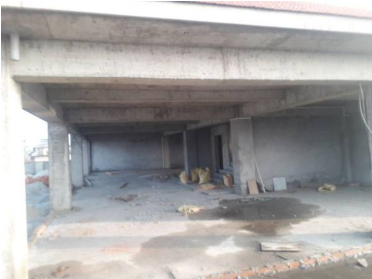
The top roof for our Solar panel :
