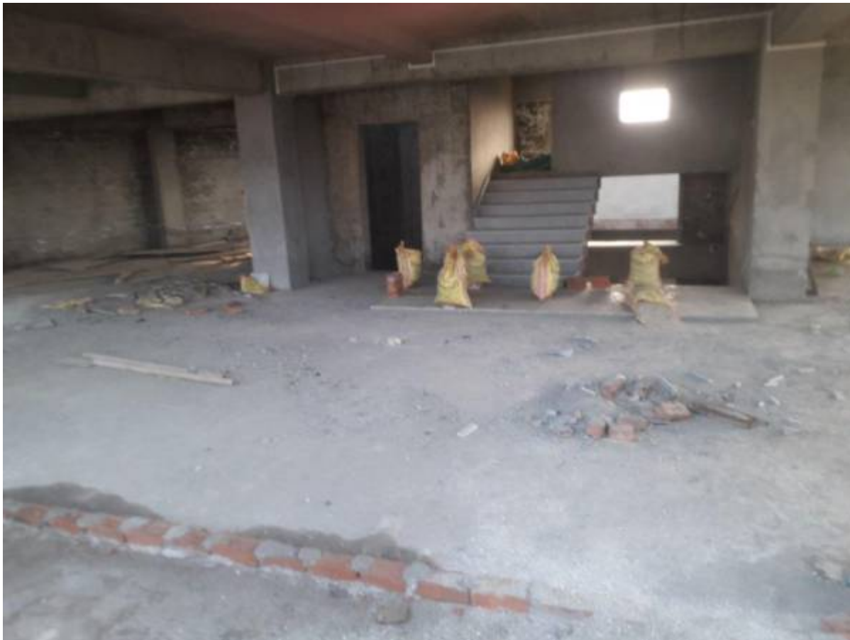
The 5ft Floor with roof access from a corner :
