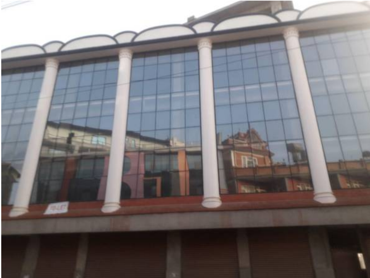
Building from the side :
