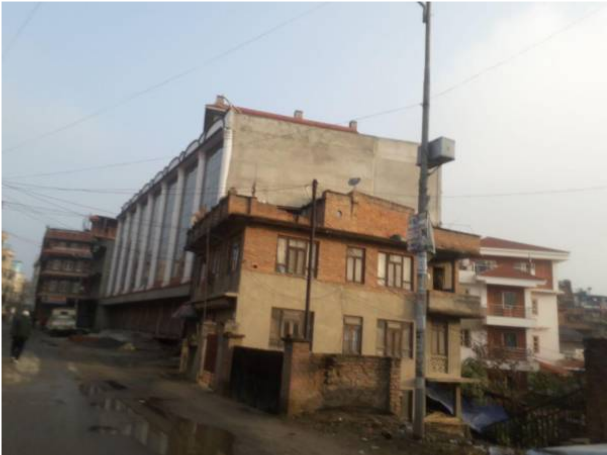
The 5ft Floor with roof access :
