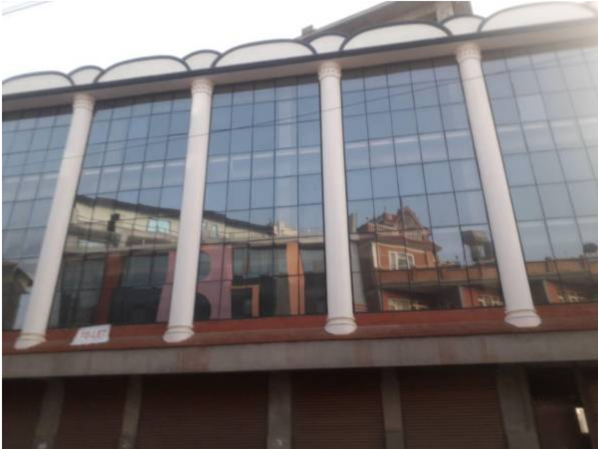
Building from the side :
