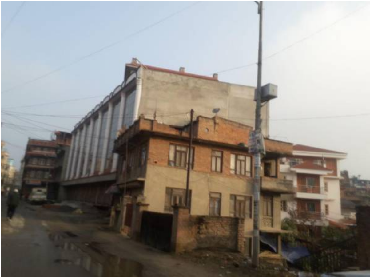
The 5ft Floor with roof access :
