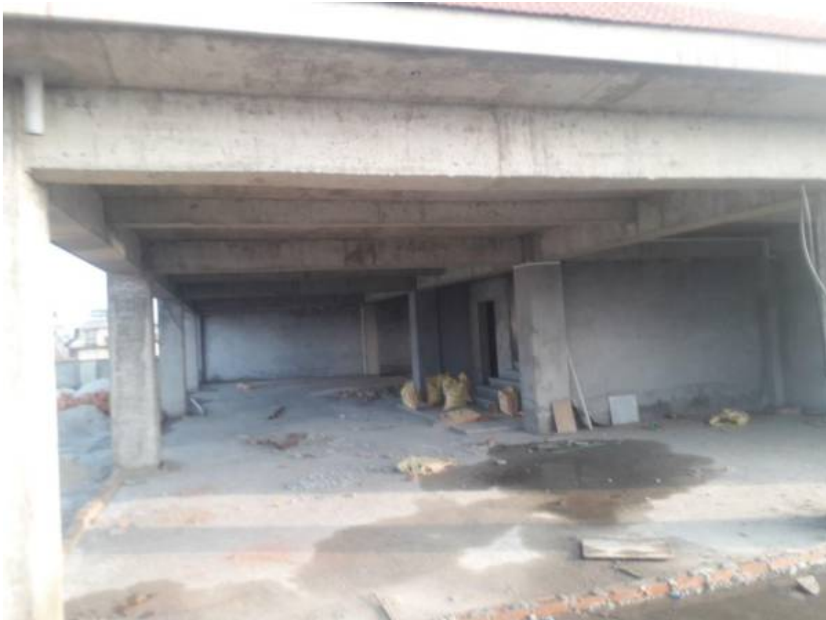
The top roof for our Solar panel :
