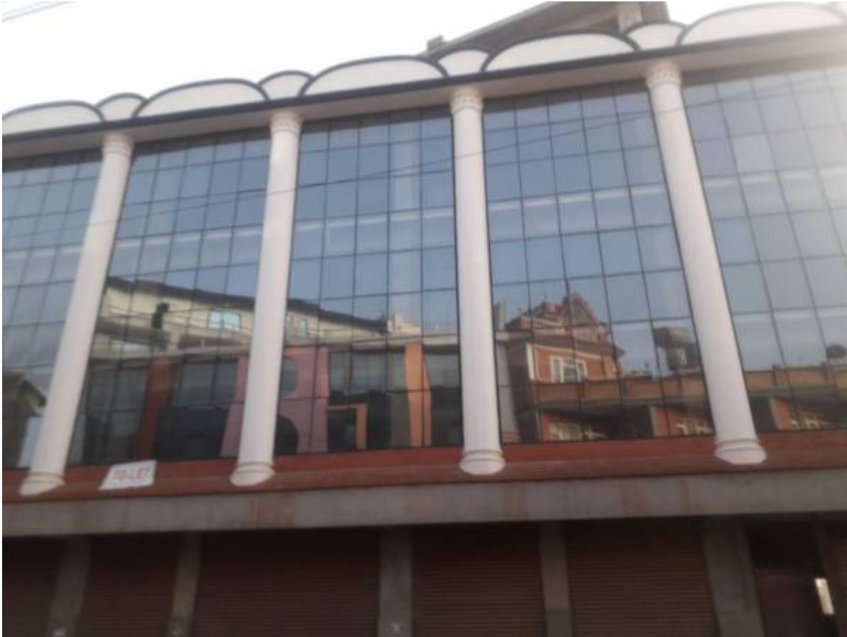
Building from the side :
