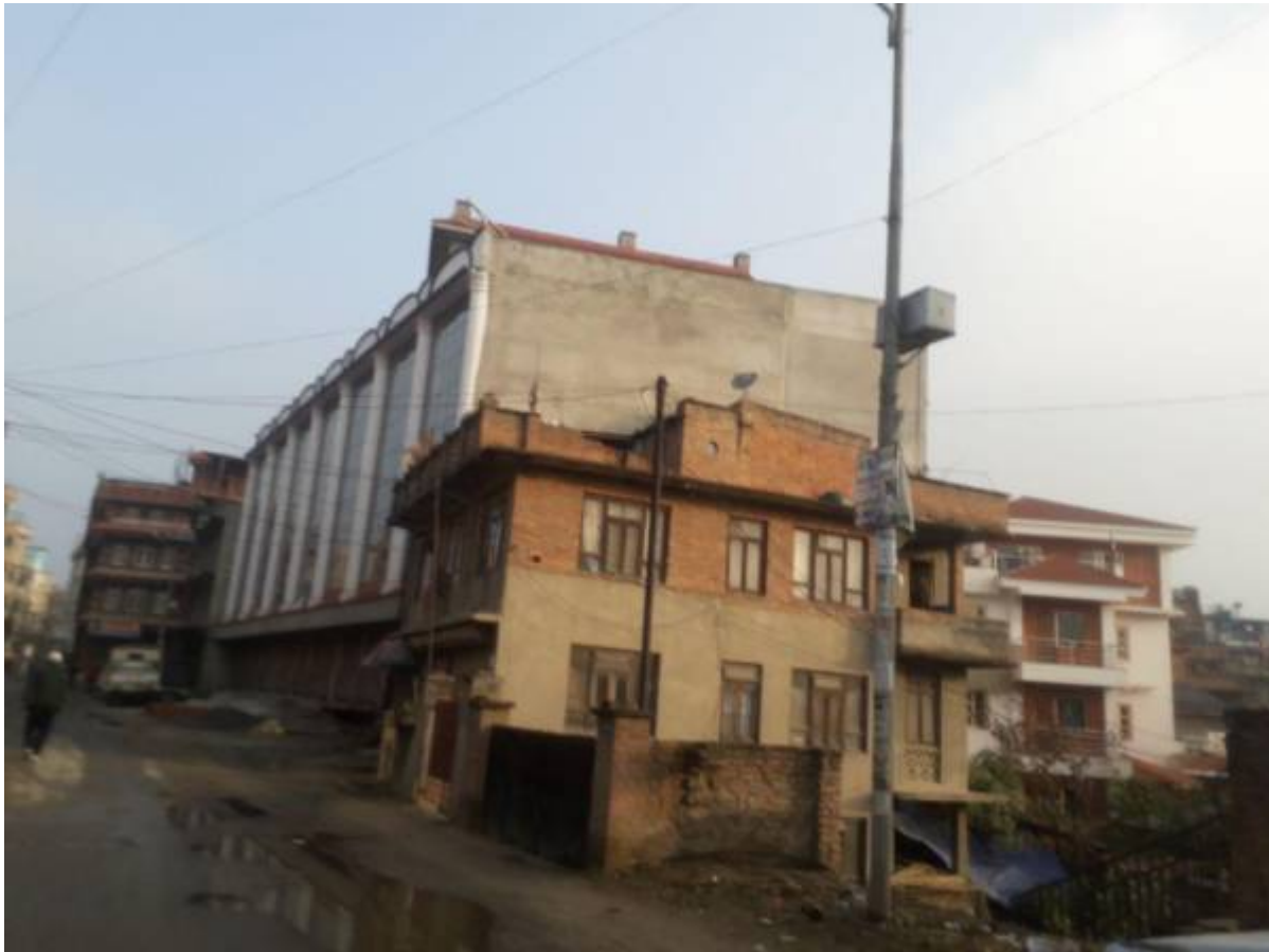
The 5ft Floor with roof access :
