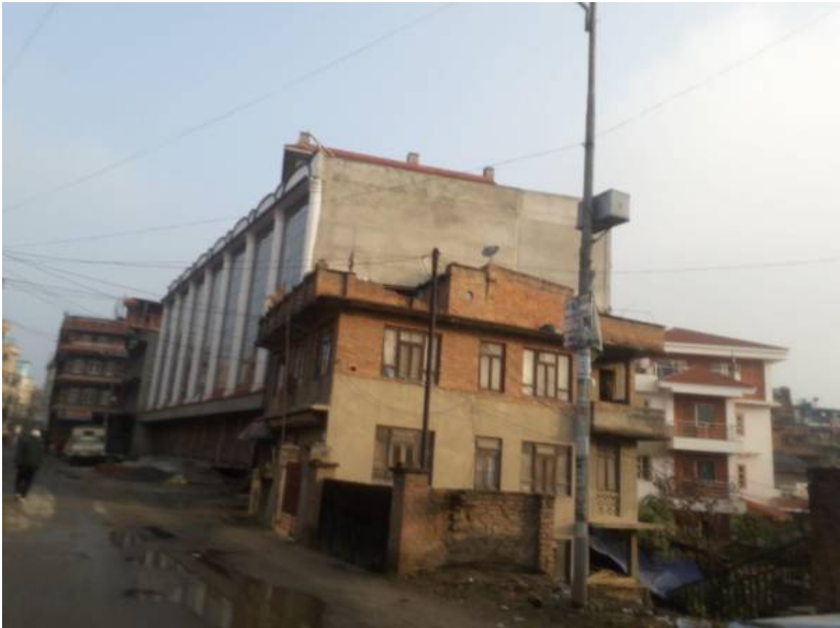
The 5ft Floor with roof access :
