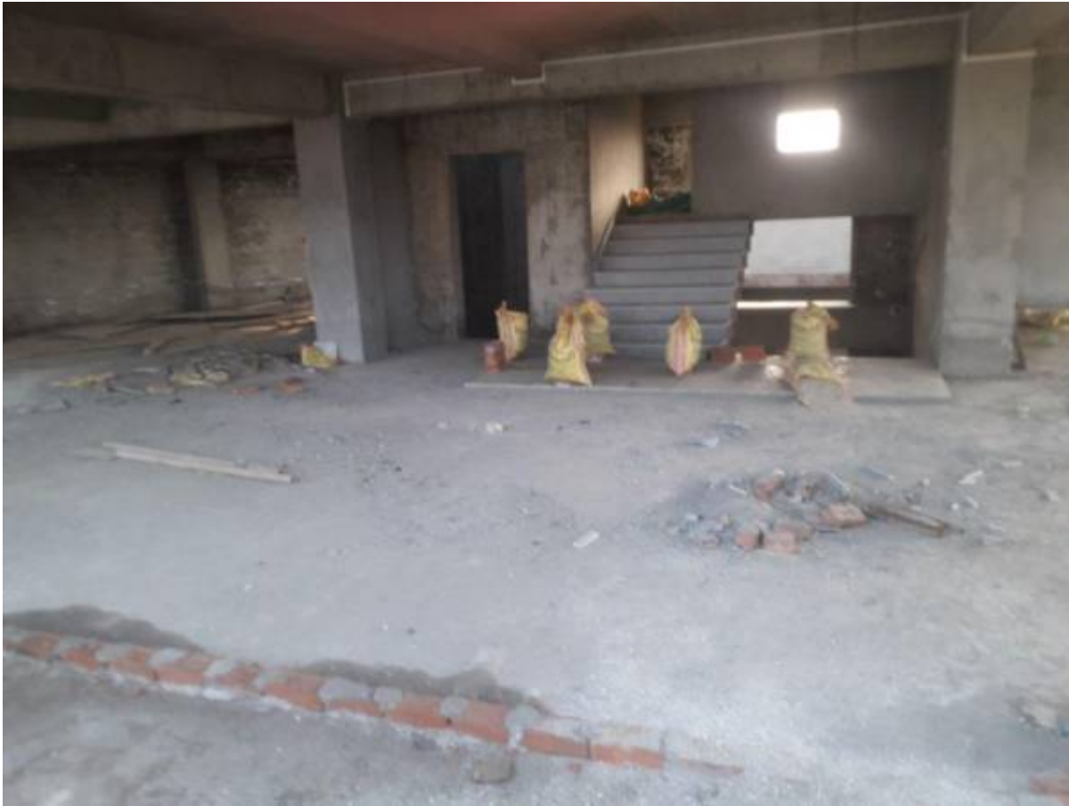
The 5th Floor with roof access from a corner :
