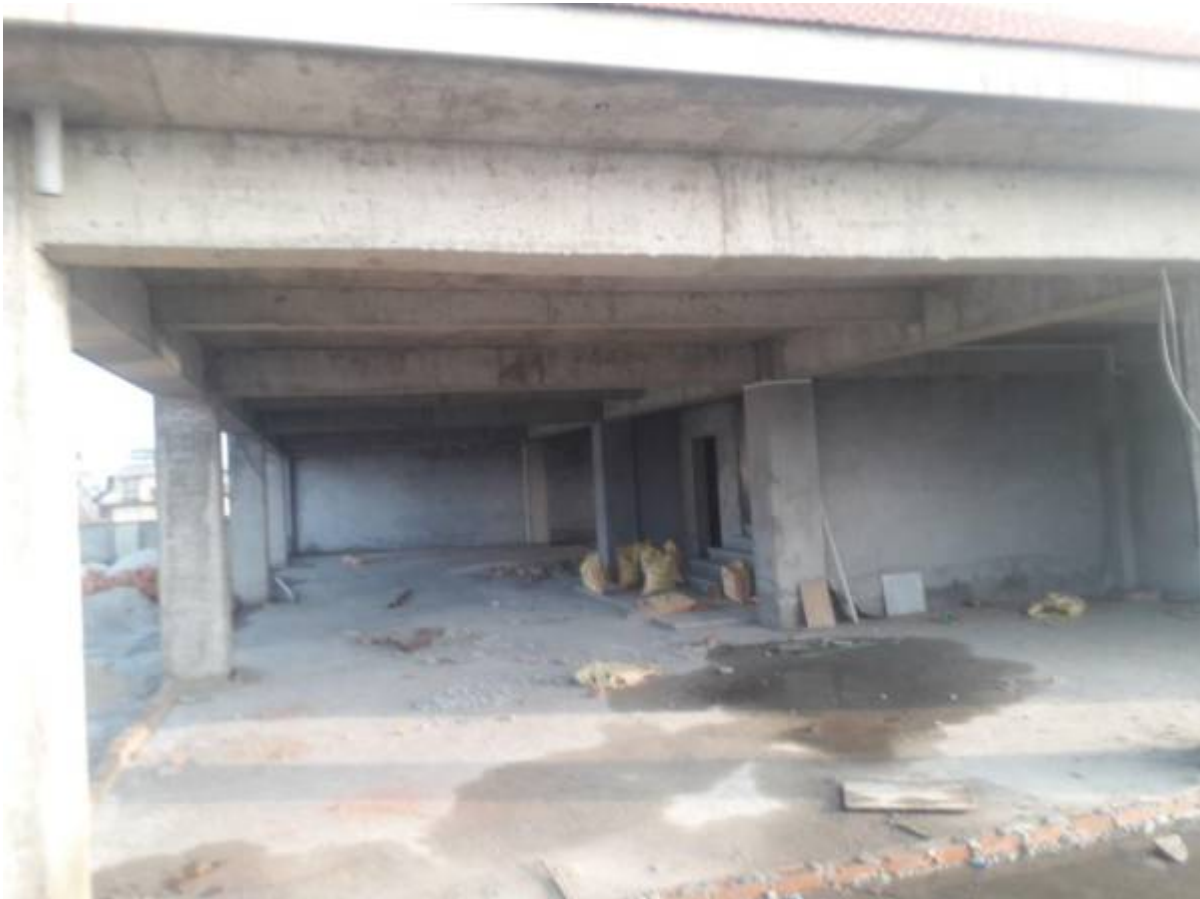
The top roof for our Solar panel :
