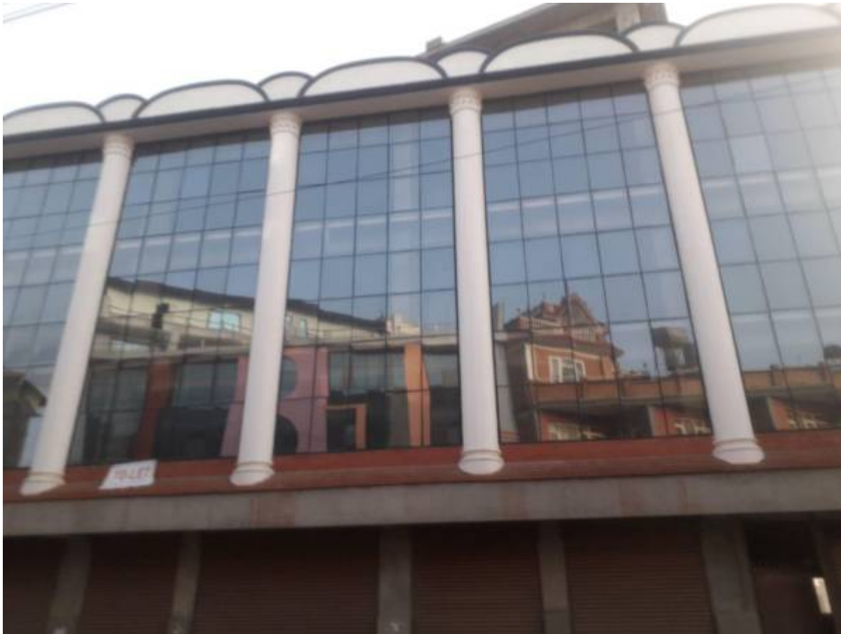
Building from the side :
